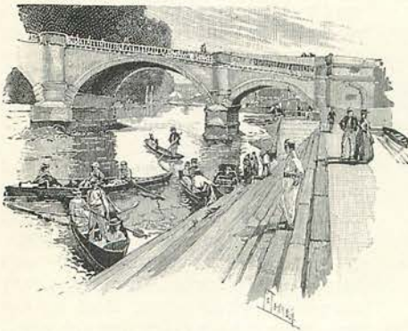
LANDING AT RICHMOND.
