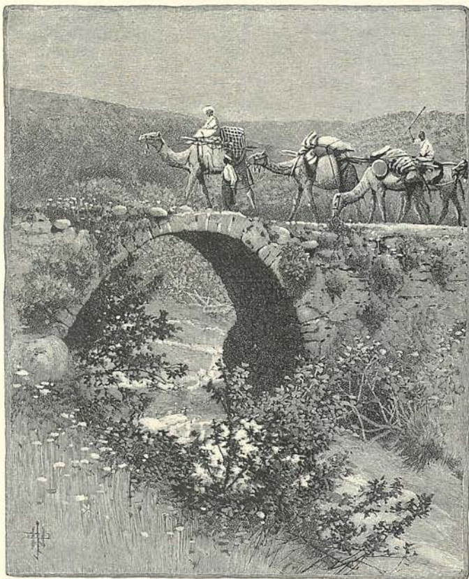
BRIDGE OVER THE HASBANY.
