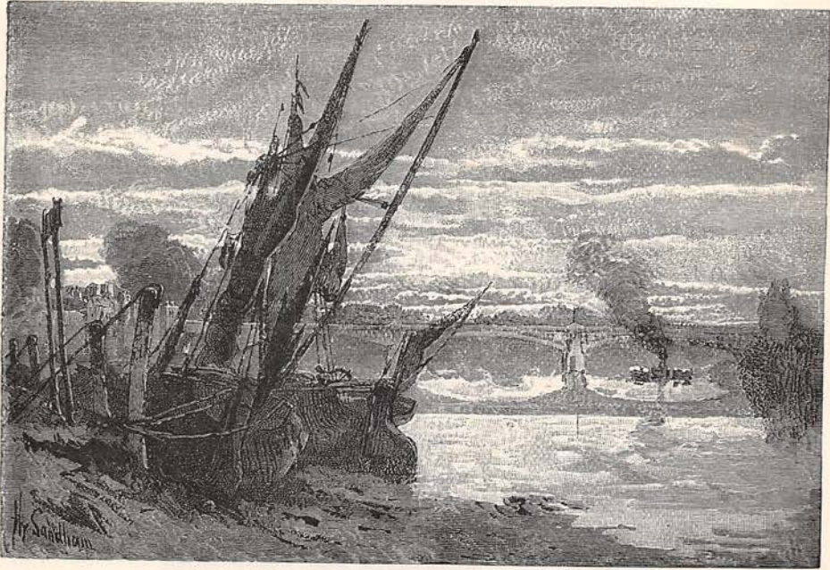
BARNES RAILROAD BRIDGE.
