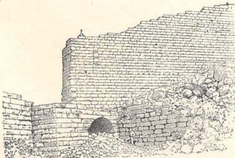
SMALL GATEWAY AND PART OF THE WESTERN TRANSVERSE WALL.
