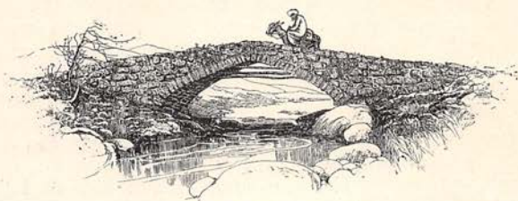
OLD BRIDGE AT GELANDEVÊK.
