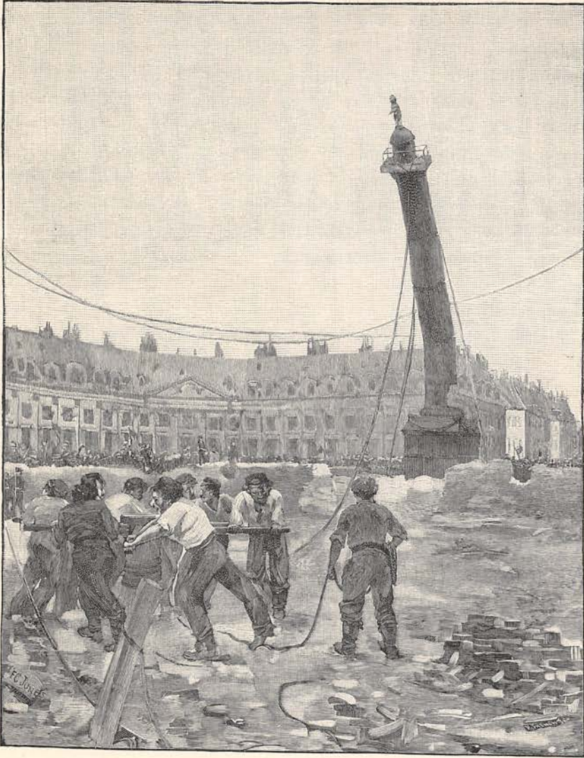
PULLING DOWN THE VENDÔME COLUMN.
