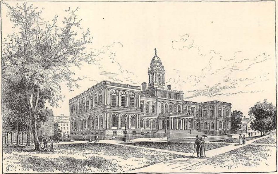
THE NEW YORK CITY HALL, FROM DRAWING BY W. G. WALL, PUBLISHED DECEMBER 20, 1826.
