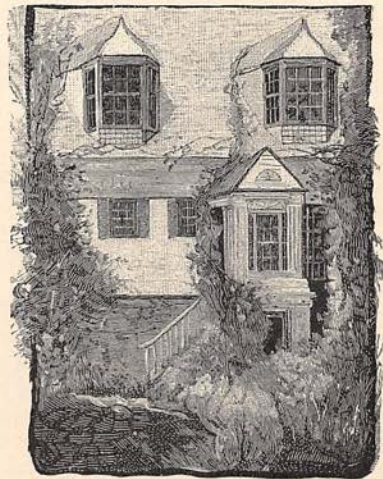
AN OLD COTTAGE AT ARICHAT.
