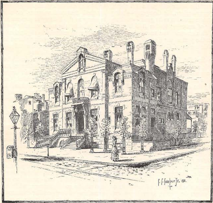
THE PRESENT BUILDING.
