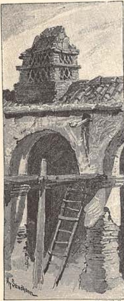
KITCHEN CHIMNEY, SAN JUAN.
