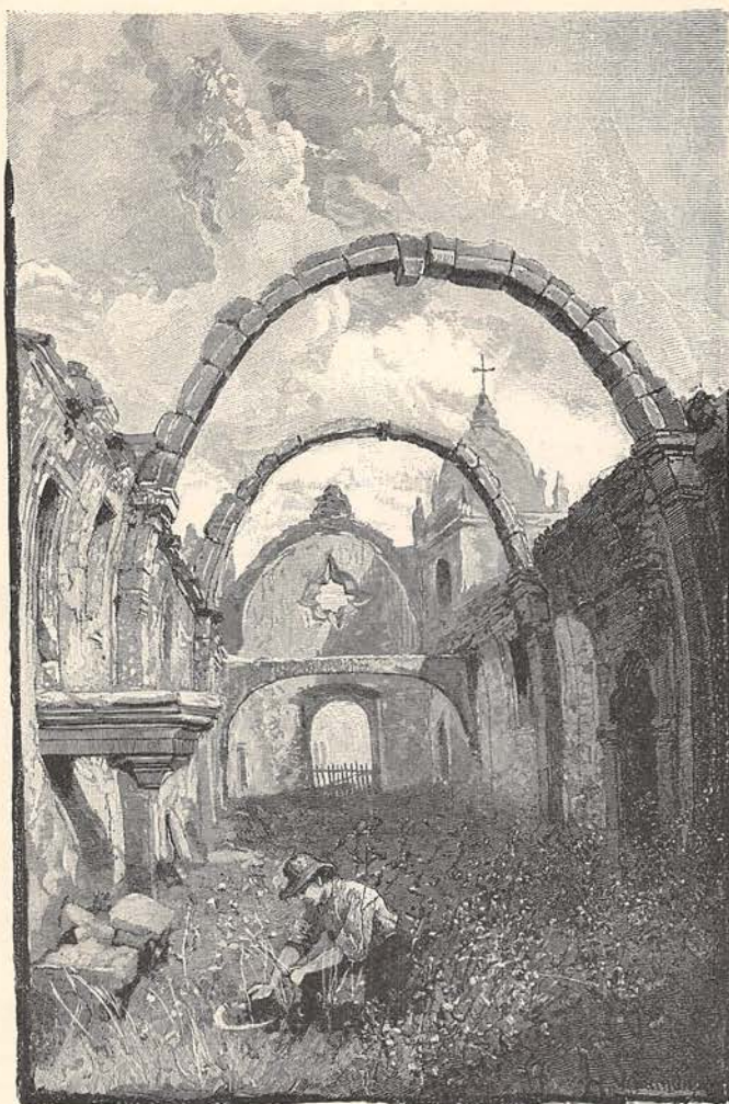
INTERIOR OF SAN CARLOS MISSION, SHOWING ORIGINAL SPRING OF ROOF AND CURVE OF WALLS.
