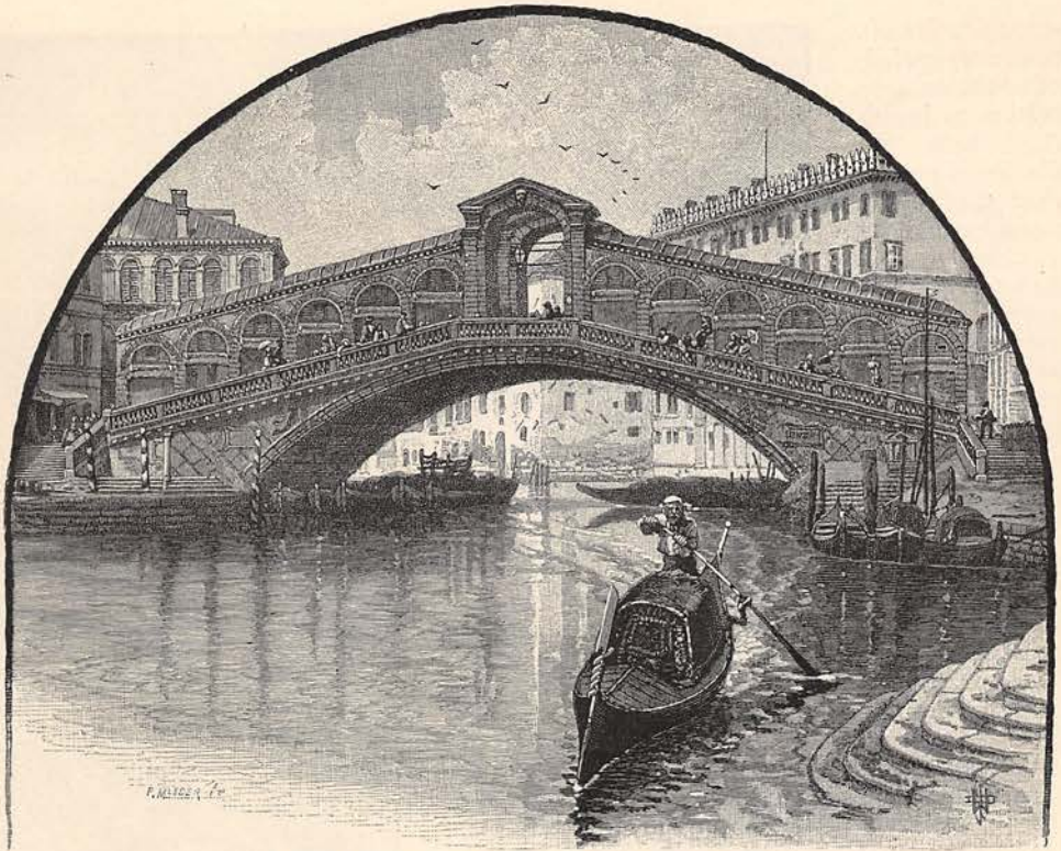
RIALTO BRIDGE, BUILT BY ANTONIO DA PONTE, 1588-91.
