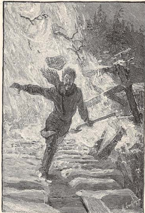
AN AVALANCHE OF SNOW DESTROYING A FLUME.
