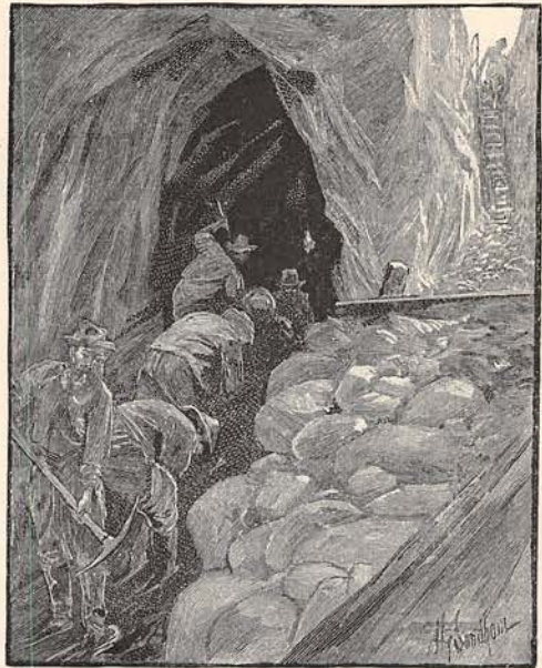
CLEARING UP A TUNNEL.
