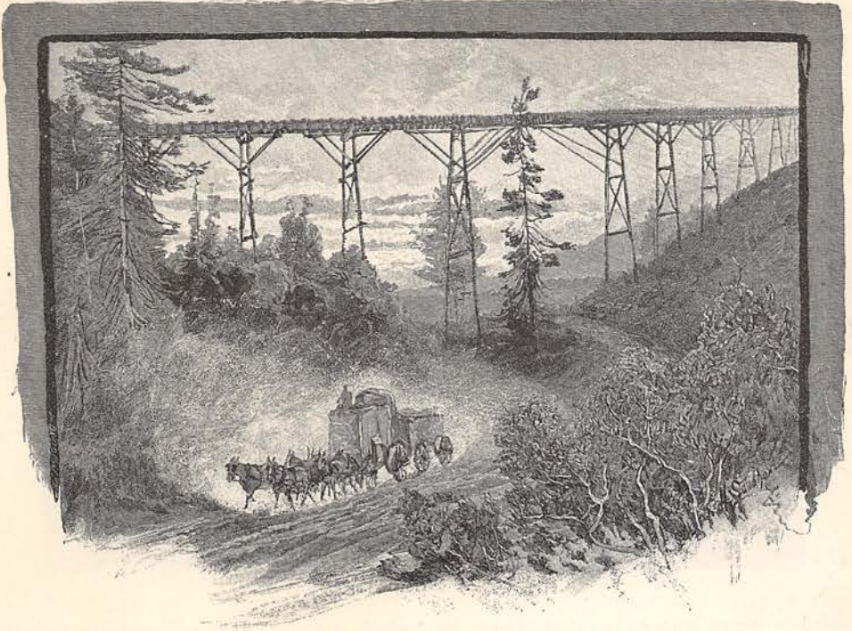
FLUME CROSSING A VALLEY.
