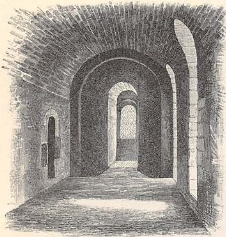
CORRIDOR IN THE TOWER, SHOWING DOOR OF RALEGH'S CELL AT THE LEFT.
