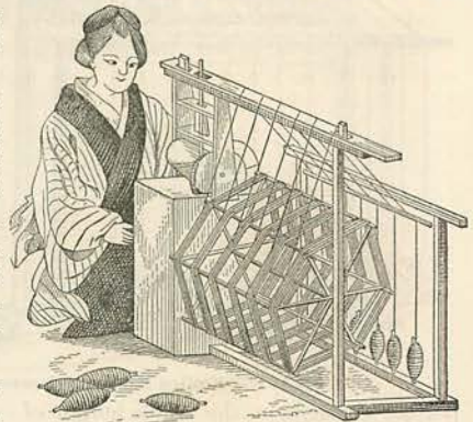
(Fig. 243.) Silk Winding Machine. Japanese Exhibit.
