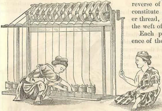
(Fig. 241.) Silk Reeling Machine. Japanese Exhibit.
